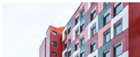
HPL RAIN SCREEN CLADDING TRESPA® METEON® ARCHITECT: CONTOR MÜLLER SCHLÜTER
