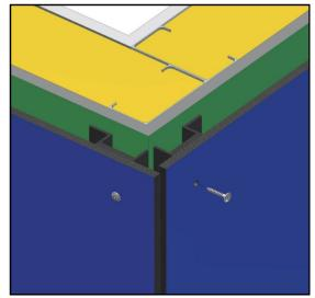
Prior to removing the clamps or blocks, drill and install at least one more fastener in the panel (for best results, choose fastener locations that will hinder the panel from shifting or rocking after the clamps or blocks are removed). When pre -drilling the substructure at the remaining oversized (larger) panel holes, use a centering tool to make sure the fasteners are centered in the hole.
